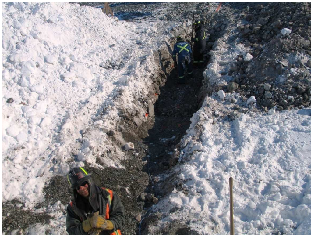
Photo 8: Sta 0+85. End of cable shown is location where it came out of the ground. Excavations in foreground were to uncover cable to where it was coiled up..
