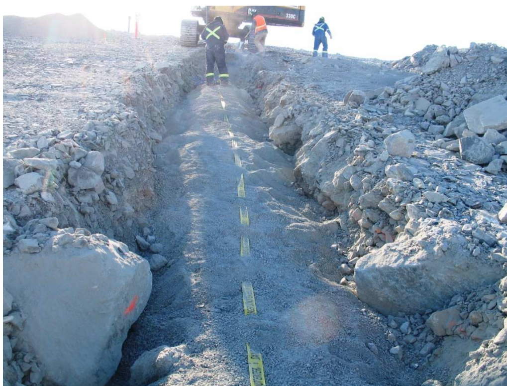
Photo 3: Sta 0+60 .6 m of crush in place. Warning tape in place.
