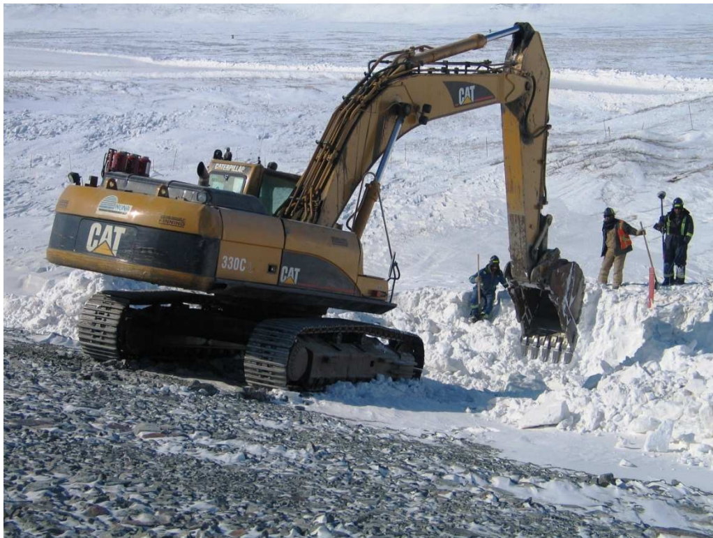
Photo 7: Sta 0+85 Locating cable. It was buried in crush .
