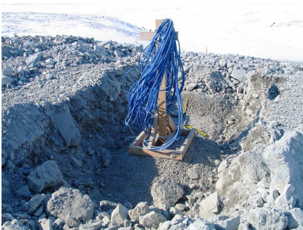
Photo 4: Sta 0+60 termination of cables
