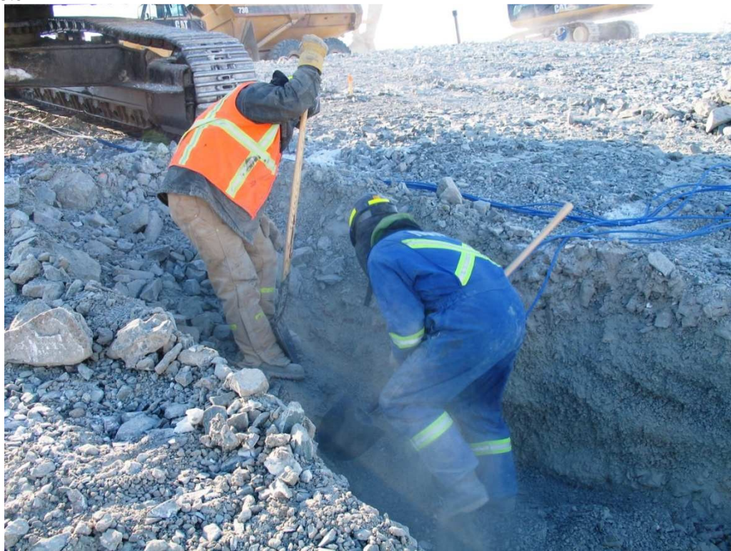
Photo 1: Stoa 0+60, excavating at cable cluster. Excavation at this point needed to be ~.5 m under the cable cluster
