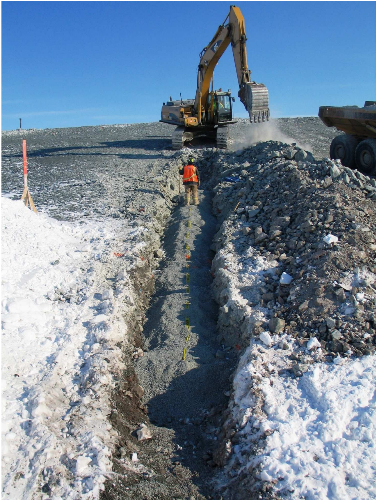
Photo 9: Sta 0+85 Progress.No buttress is planned as there is adequate cover.
