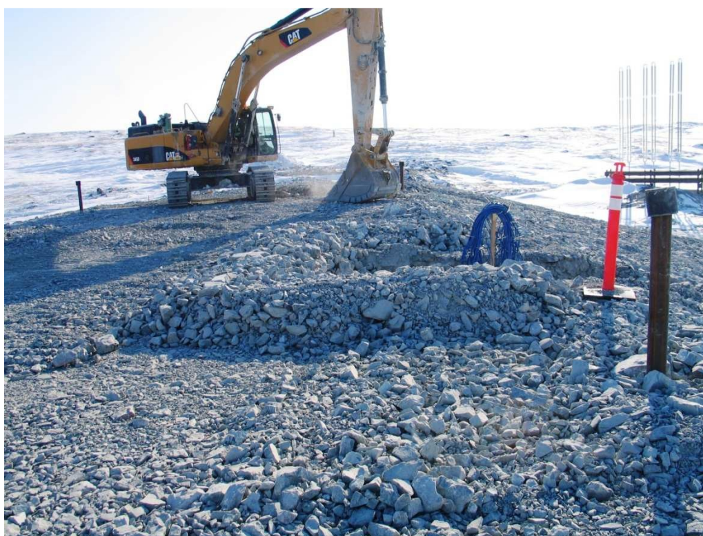
Photo 6: St 0+60 Safety berm at ermination point.
