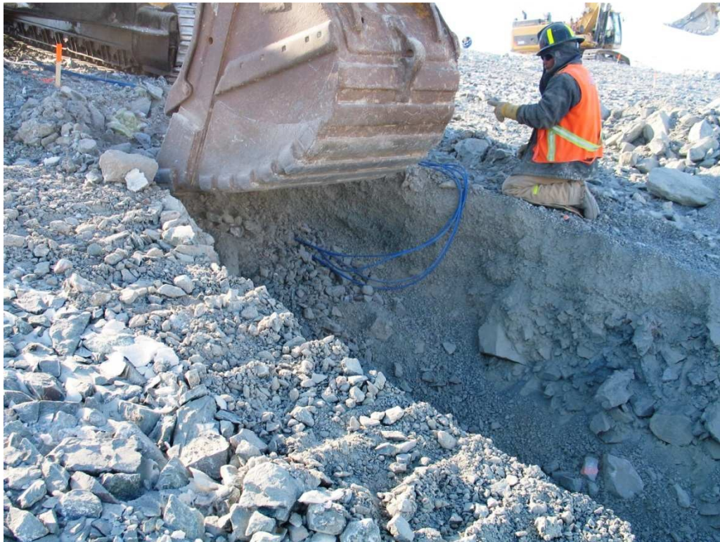
Photo 1: Stoa 0+60, excavating at cable cluster. Excavation at this point needed to be ~.5 m under the cable cluster
